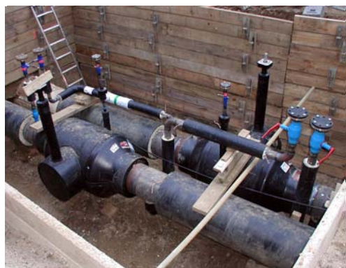
Ballostar ball valves pre-insulated, shown before and during the installation into a district heating network
