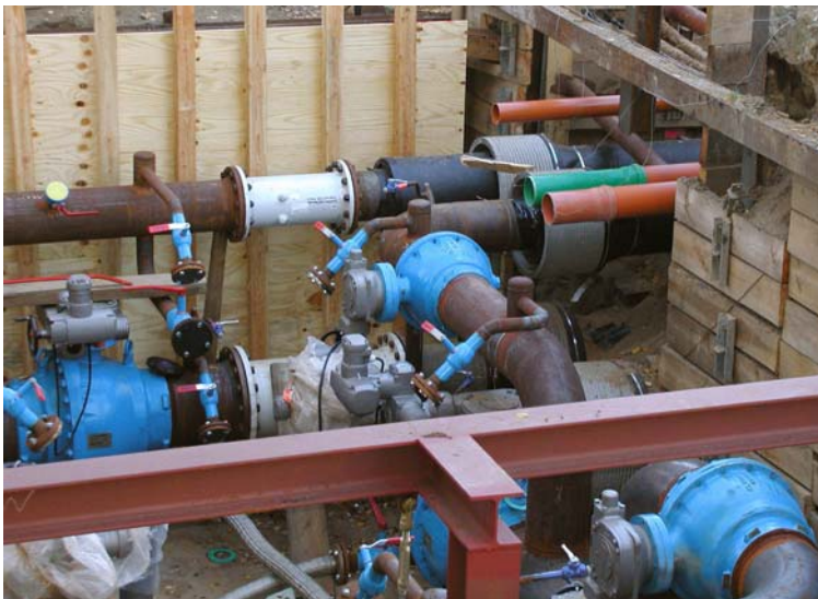
Installation site of Stadtwerke Kiel (Kiel's municipal utility): KLINGER Ballostar KHSVI and Monoball ball valves
