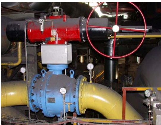
KHI DN 400 equipped with pneumatic actuator
